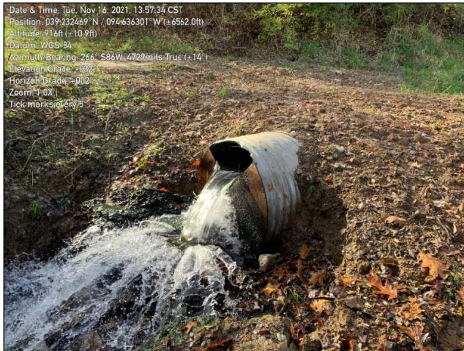
Figure 4- West Abutment Seepage Weir
