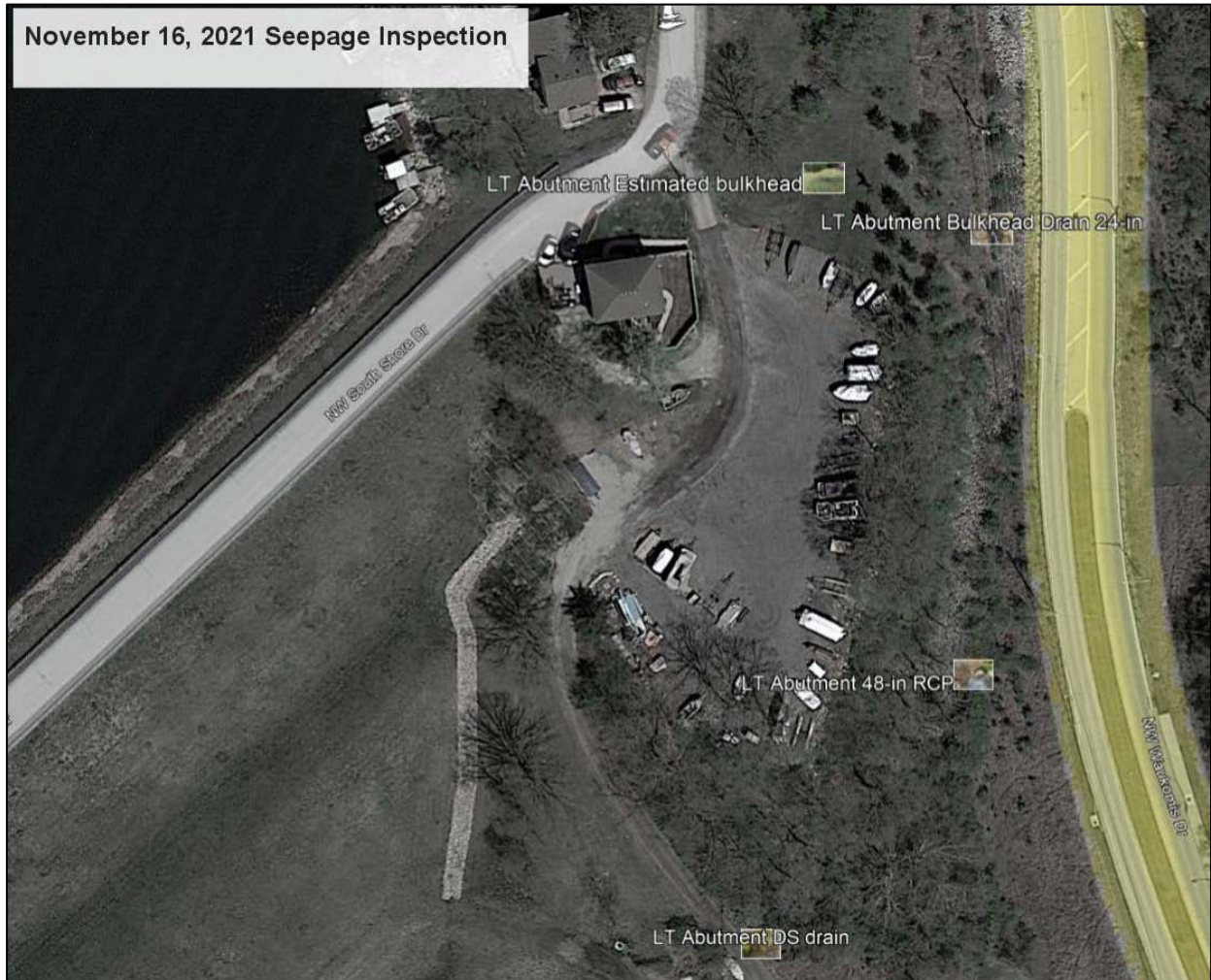
Figure 5- East Abutment Seepage Location
