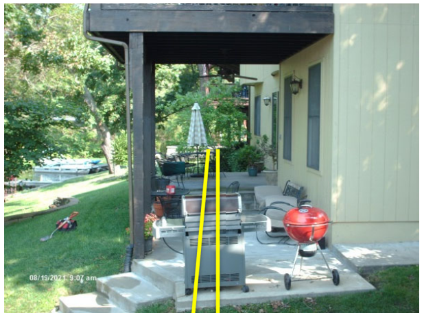
Sewer runs below patios and decks. Hopefully excavation not required....
