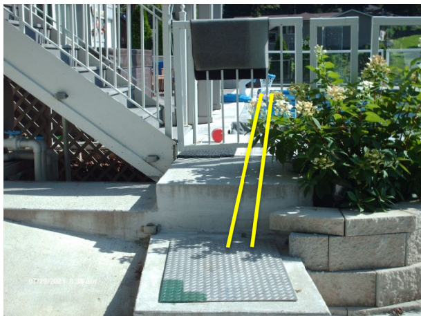
Sewer line under pool. Manhole under deck and wall. Repairs will be interesting...
