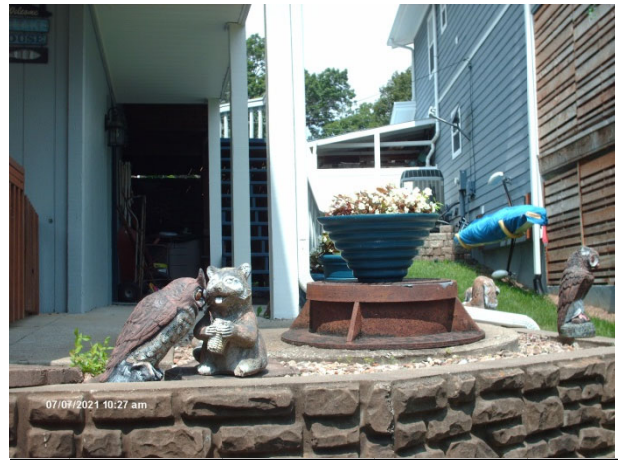
Manhole surrounded by walls, landscaping. Difficult access.
