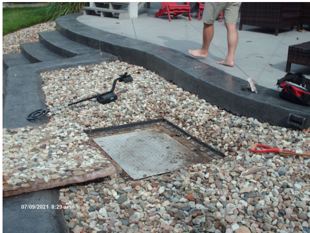
Ingenious camo'd cover by homeowner, rocks glued to board... But new MH needed, raised to grade.
