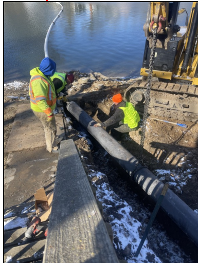
The new siphon line is installed between the 800 and 900 blocks. Photos courtesy of Jack Williams and Rick Zelfer.
